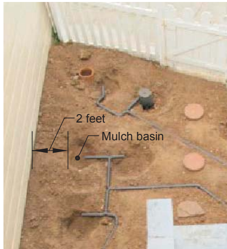
Sample image of a graywater system pre-burial. Photo: Josh Lowe.
