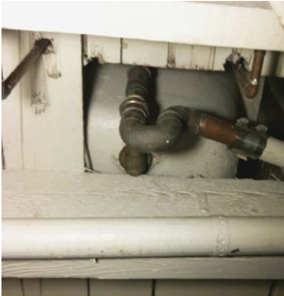
The shower p-trap is the copper pipe shaped like an upsidedown and sideways letter "p." In this example, the p-trap and shower drainage pipes are located below the shower/tub. Photo: Josh Lowe.
