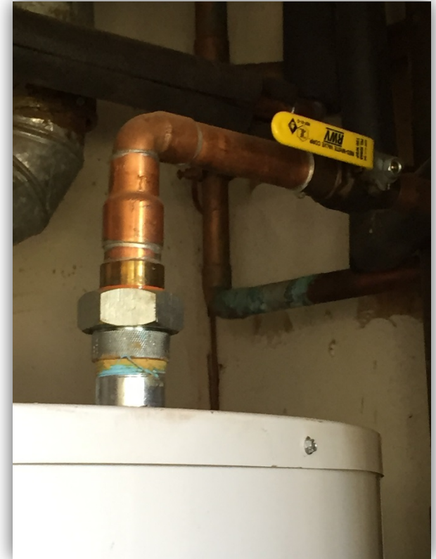
Corroded hot water piping
