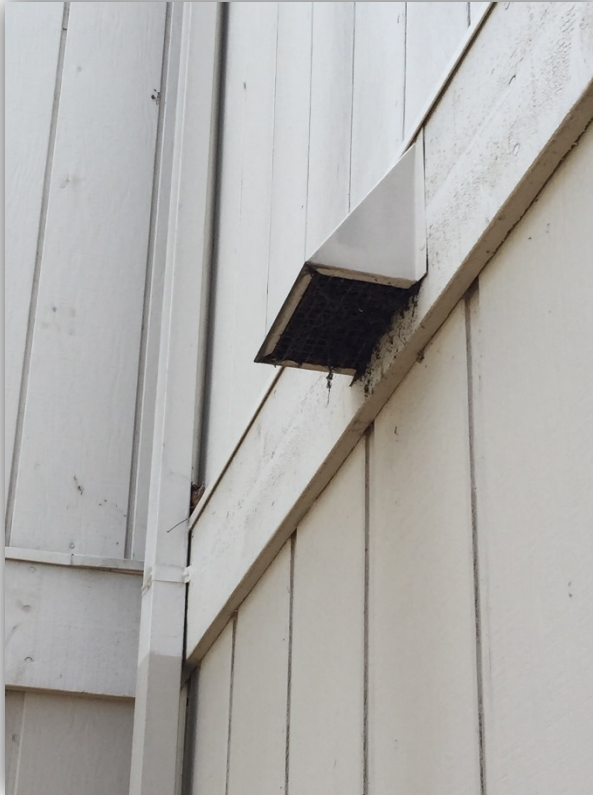
Blocked dryer and range hood vent
